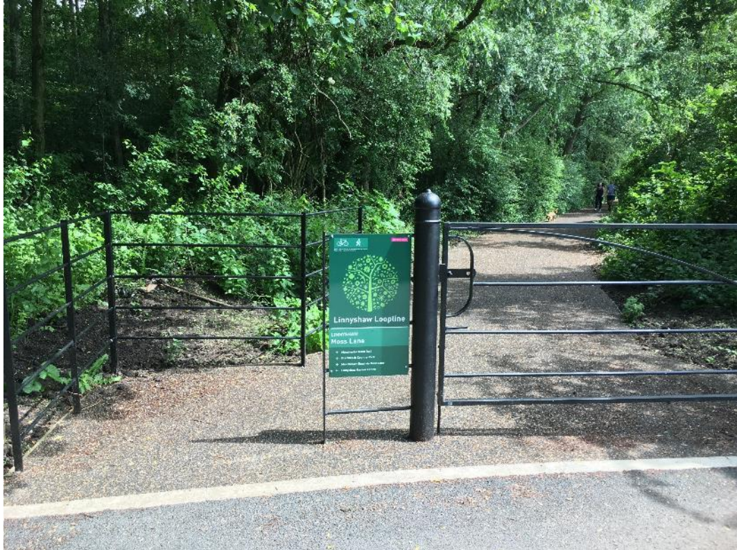
Figure 3: Accessible access control gate with lockable access for maintenance vehicles, Linnyslaw Loopline, Salford
