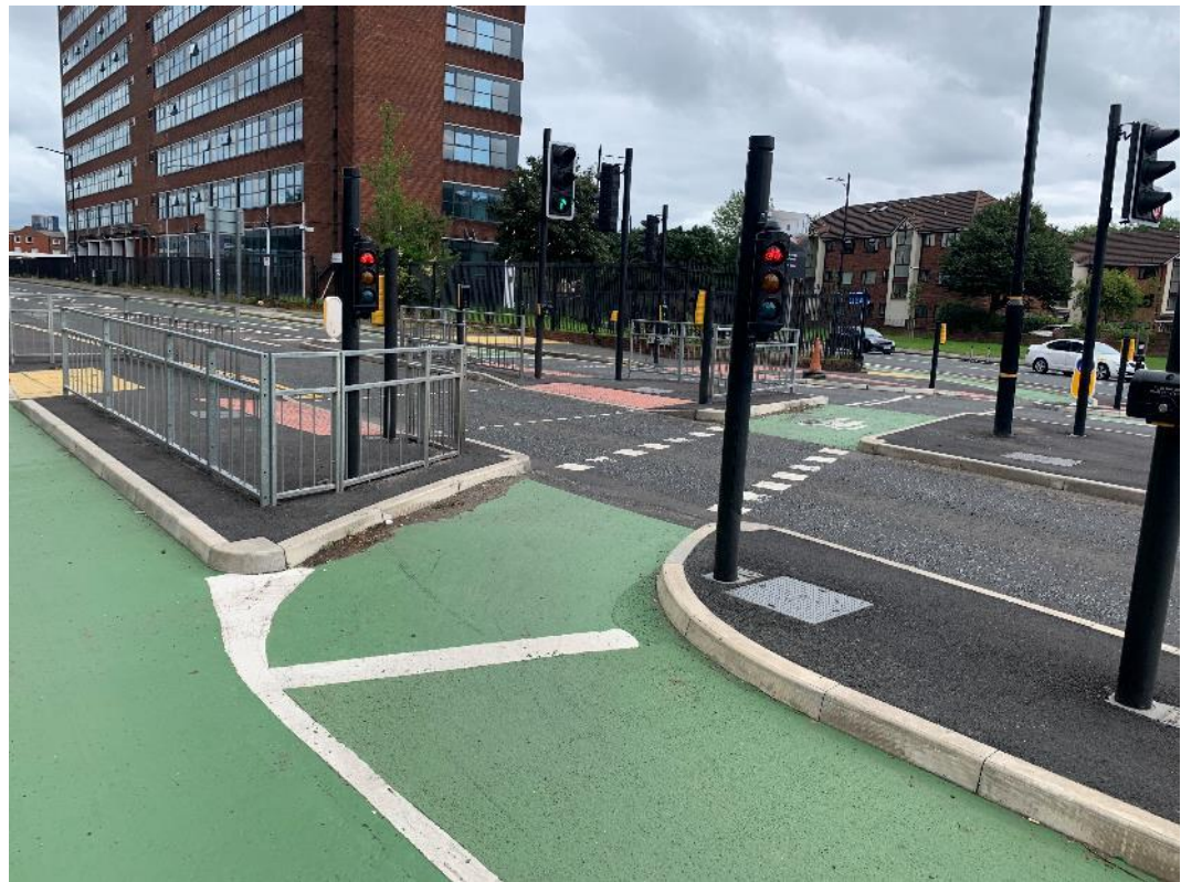
Figure 14: Protected right turn dedicated cycle phase, Trafford
