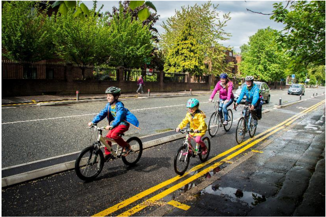
Figure 1: Example of protected cycle provision on a busy road: kerb protected cycle lane in Fallowfield (Manchester)
