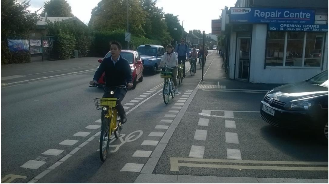
Figure 16: Side road with marked priority for cyclists and pedestrians, Walthamstow
